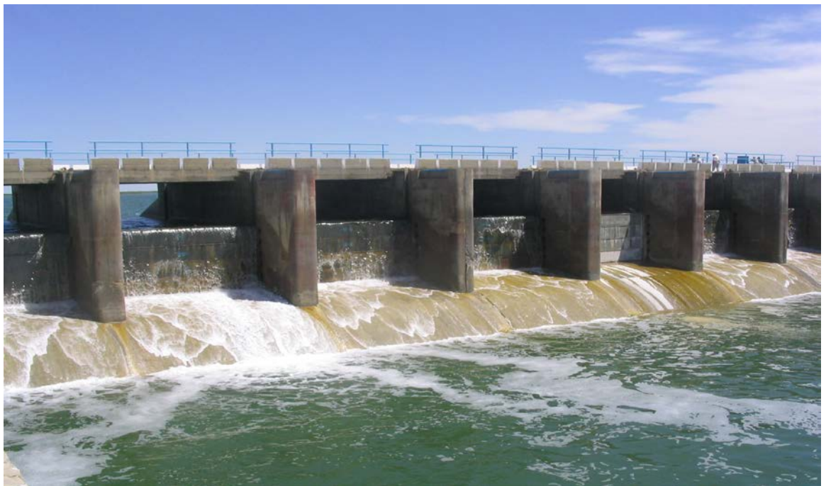
Fig.A2. Spillway at NAS dam.
