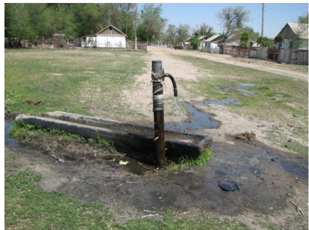
Remains of old potable water system in a Kazakh village
