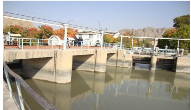
Isfara river headwork
