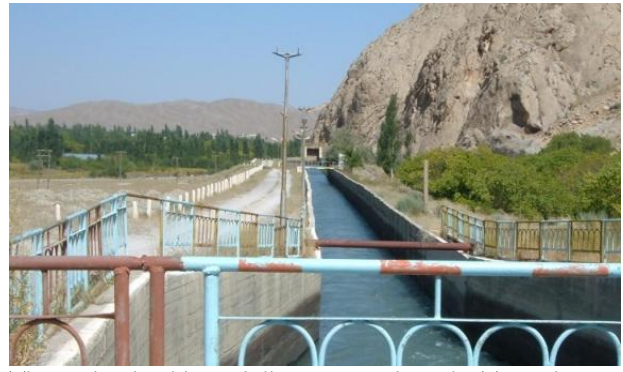
The Podvodyashi canal diverts water into the Tortgul reservoir
