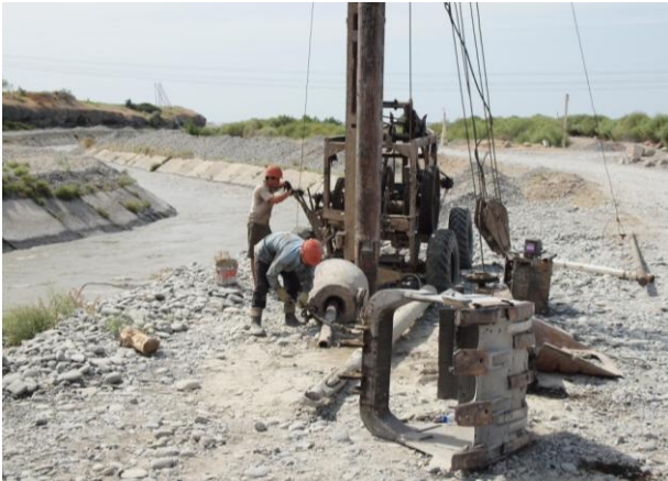
Groundwater observation bore at Ravatkhodja headwork
