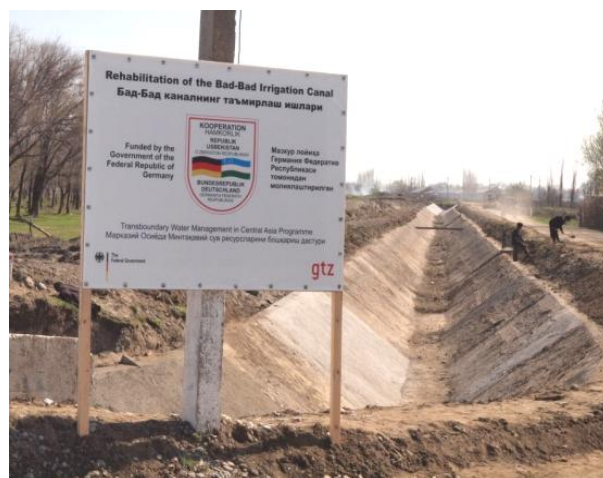
Rehabilitation works at the canal
