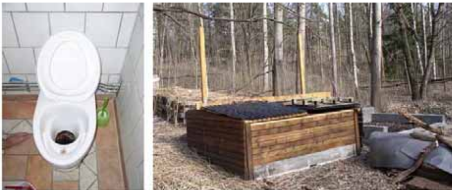
Figure 14. (left) The sanitation system is unique: a urine-diverting system with dry collection of faeces in a 2-storey building. Photo: Mats Johansson.
