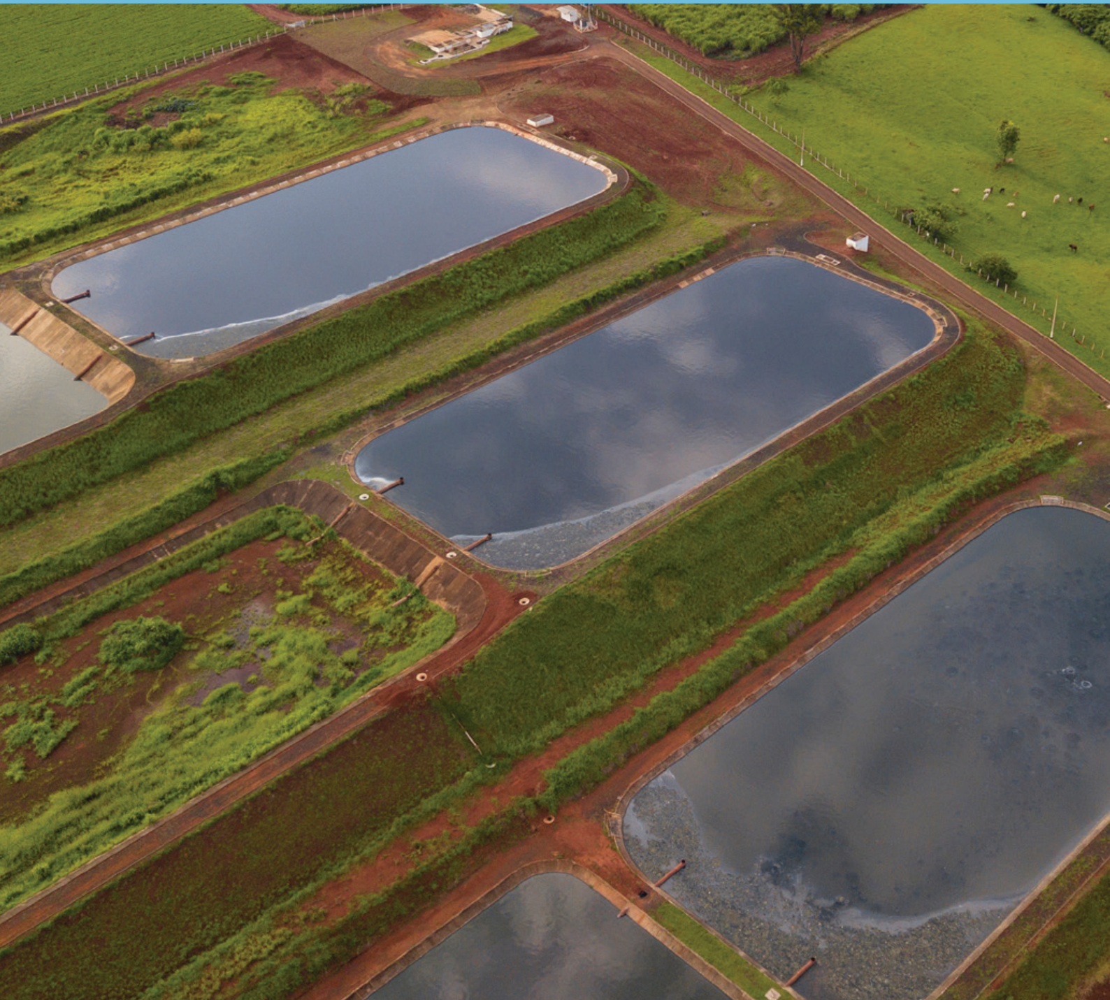
Aerial view of a sewage treatment facility.
