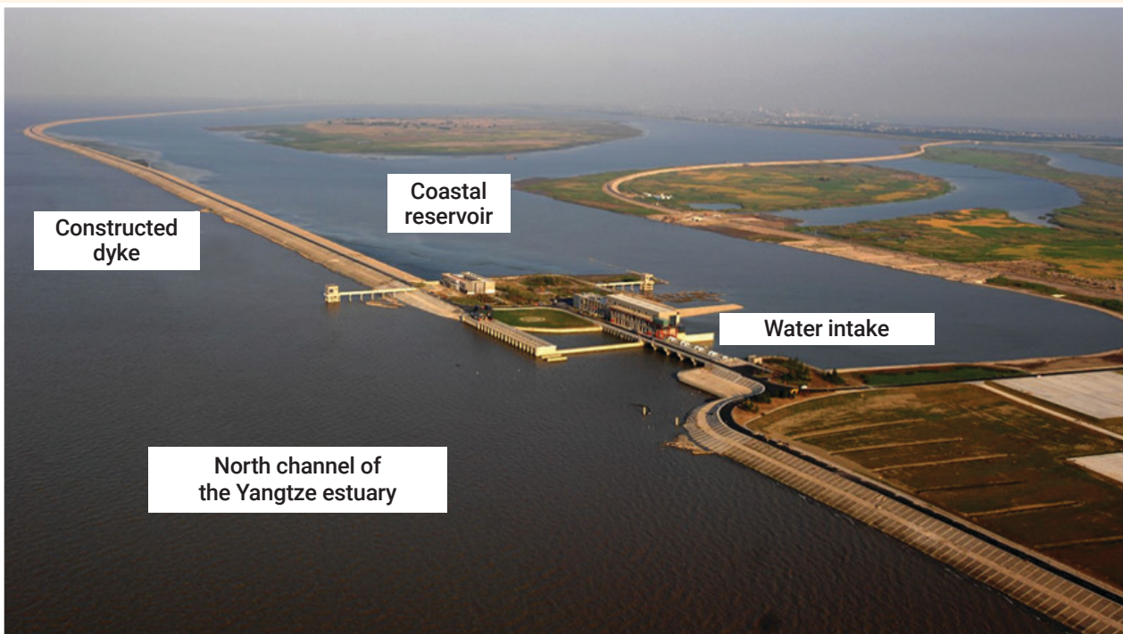
Figure Aerial view of the Qingcaosha Coastal Reservoir at the mouth of the Yangtze River
