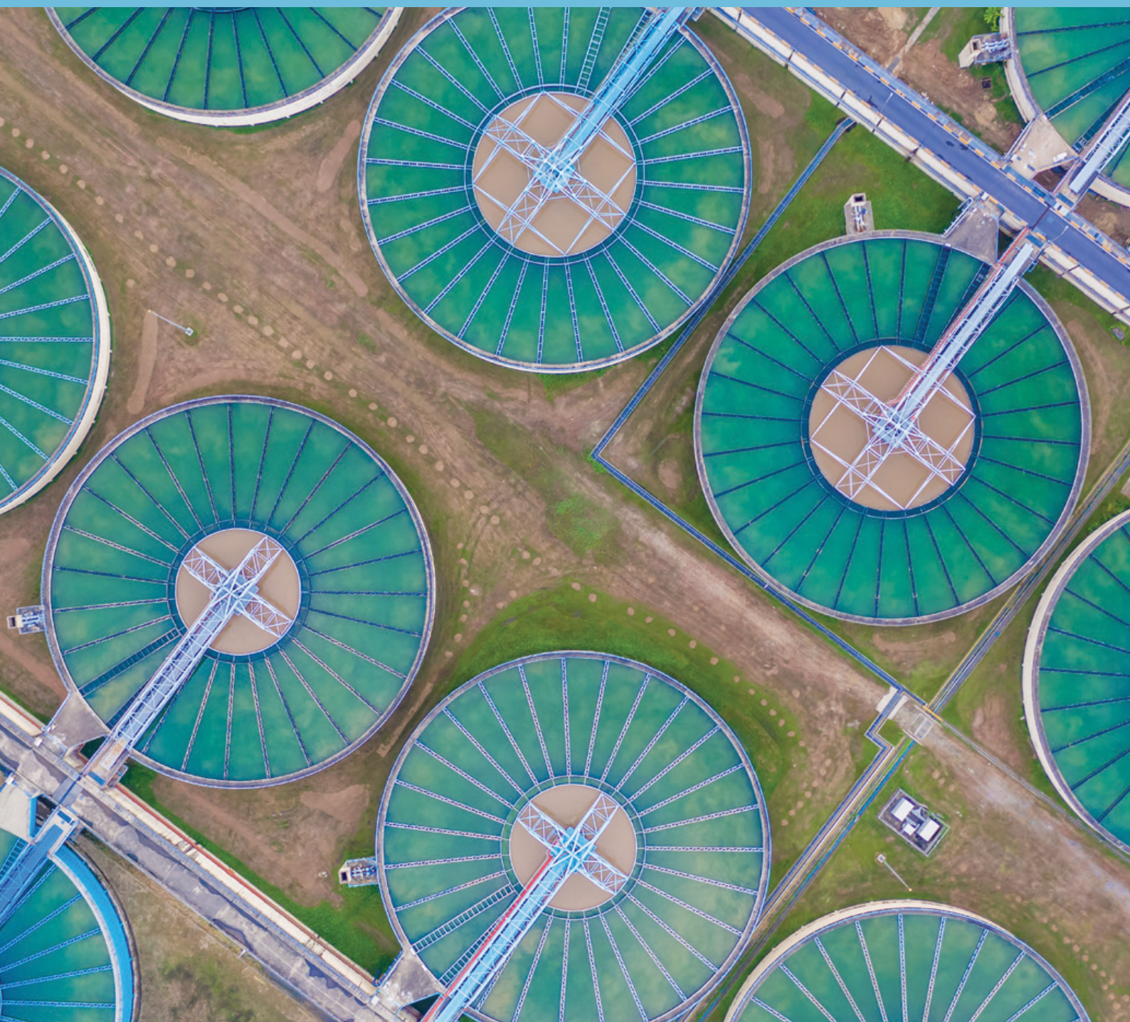
Aerial view of a water treatment plant.
