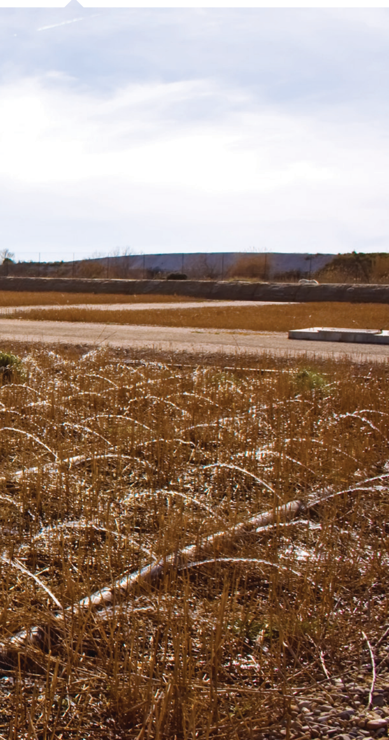
Constructed wetlands for wastewater treatment plant
