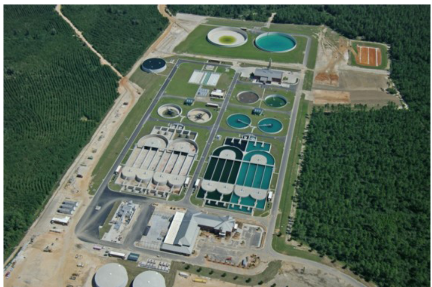
The wastewater treatment plant in Escambia County, Florida (USA), destroyed by Hurricane Ivan, and replaced and relocated away from the coastal plain and built to be more resilient. The plant now reuses 100% of its water.
