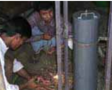
Arsenic Removal Family Filter being set up in a Bangladeshi home
