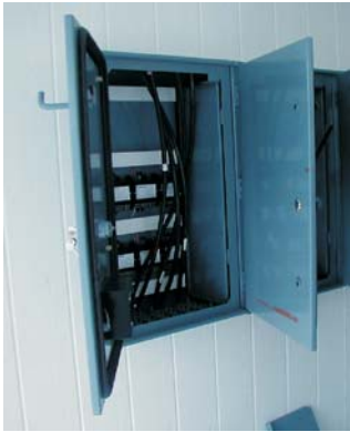
Fig. 4. Cupboard for controllers and input and output modules
