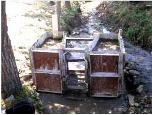
a) On-site manufacturing flumes using collapsible portable formwork
