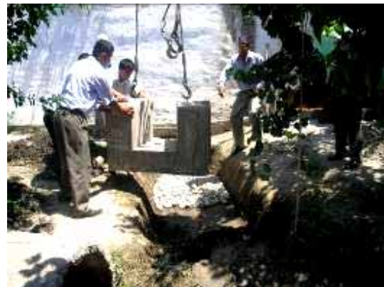
b) Assembling pre-cast flumes
