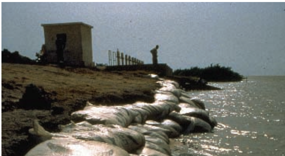
Sandbags along river dike in Senegal river delta, Mauritania
