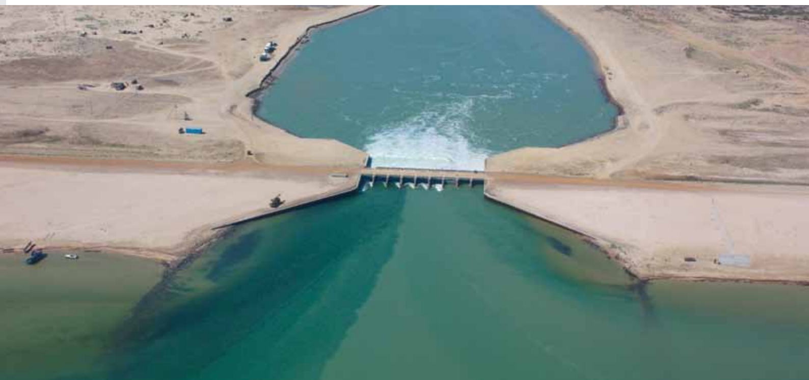
The Kokaral dam spillway
