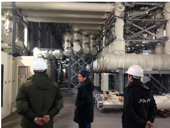
Indoor switchgears
