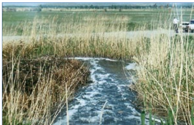
Pic. 9. Discharge of effluents to the filtration fields in Taraz town (Kazakhstan)
