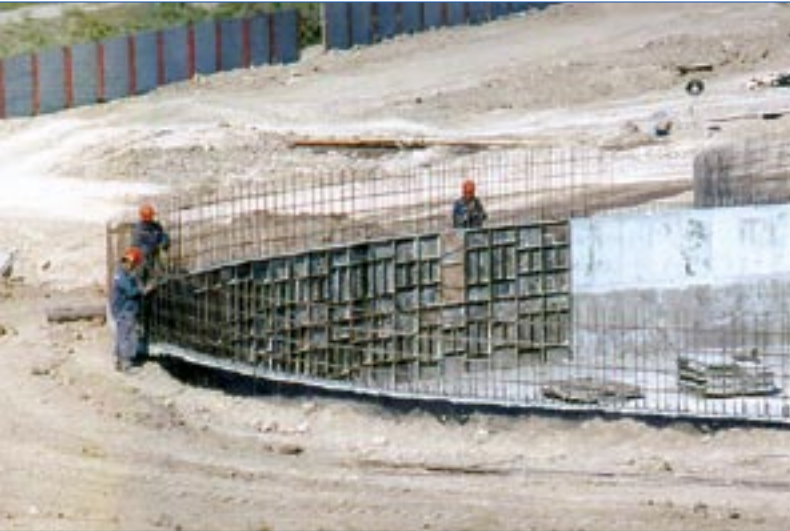
Pic. 13 Construction site of station for biological rectification in Kyzylorda (Kazakhstan)
