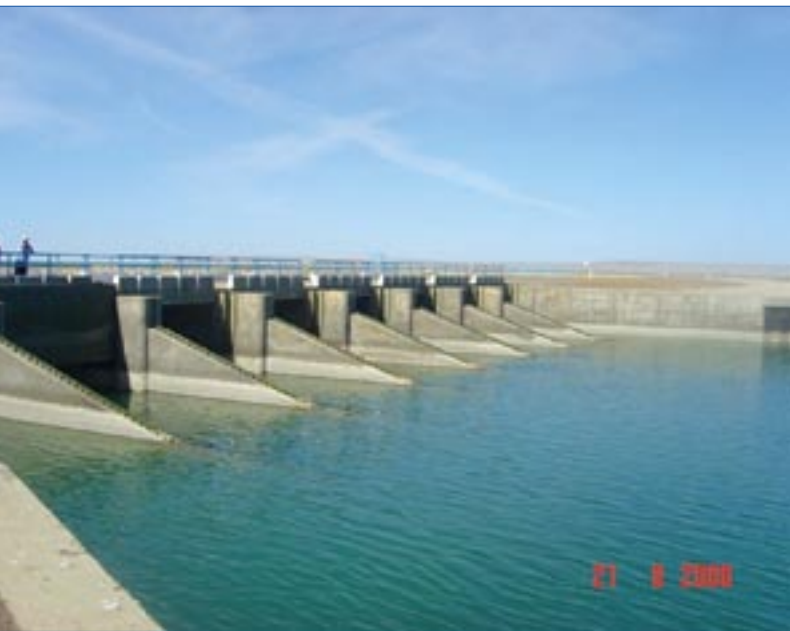
Pic. 14. Hydro-technical complex on Kokaralskaya dam in the Small Aral (Kazakhstan)
