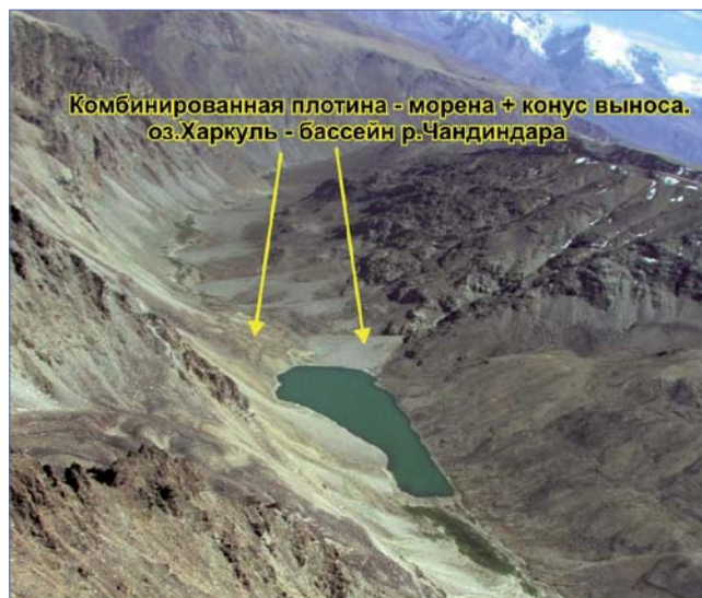
Photo 20. A composite dike at the Kharkul Lake
