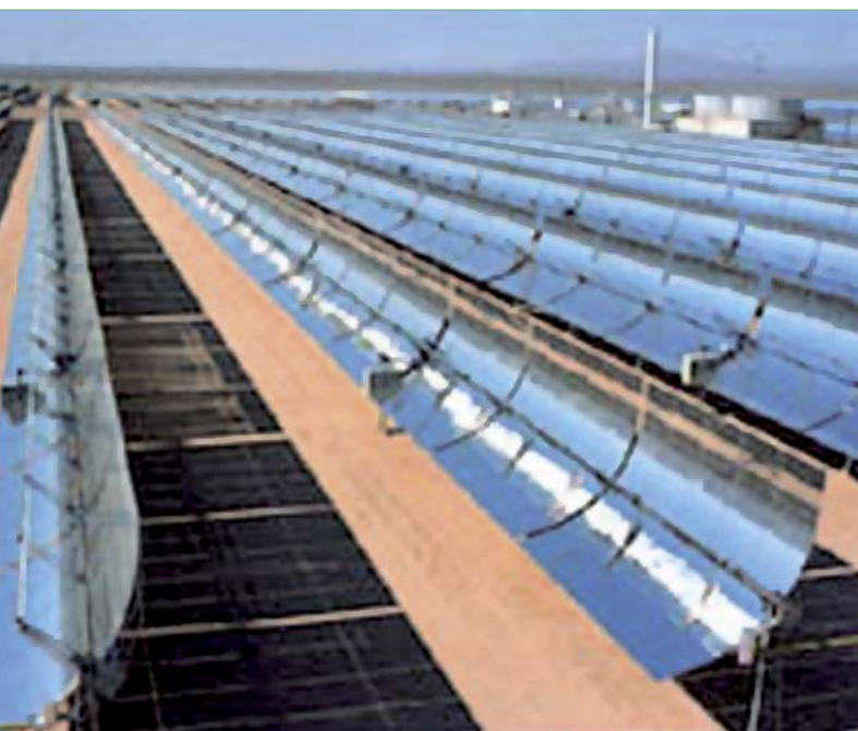
Fig. 3. Solar power plants
