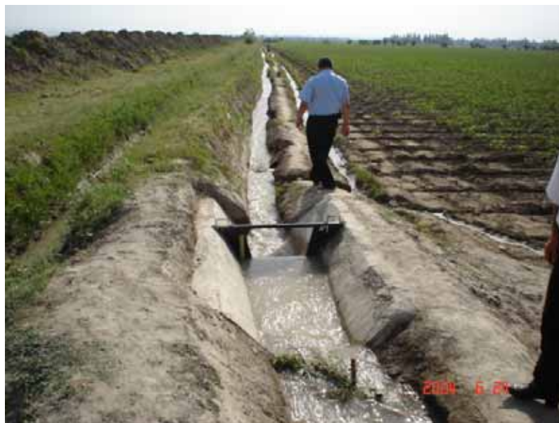
Figure 15. Water-metering weir at farmer's inlet in the WUA "Zarafshan", Tajikistan (the photo made by V. Sokolov)
