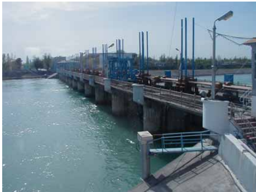
Figure 14. The Uchkurgan Hydroscheme on the Naryn River equipped with the SCADA system within the project financed by the SDC (the photo made by G. Poltarev)
