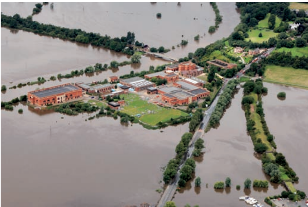
Flooded drinking-water treatment plant Gloucestershire 2007 (United Kingdom)
