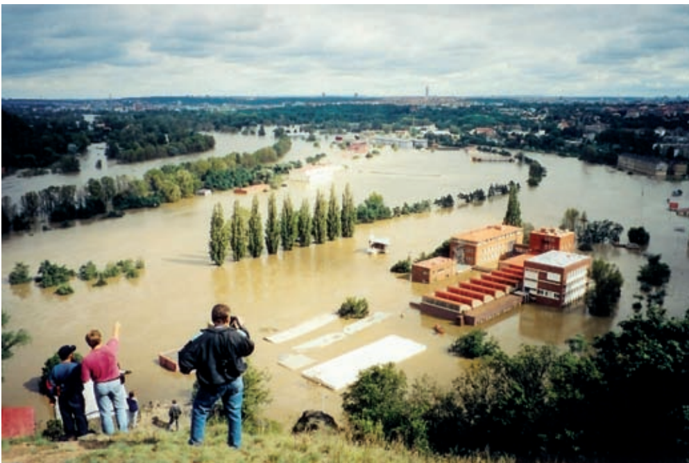
Flooding of urban wastewater treatment plant, Prague, Czech Republic (2002)
