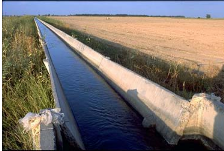
Fig 3. An irrigation canal in Hunger Steppe.
