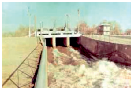
Feeding structure at 42 km of the Shavat branch's canal
