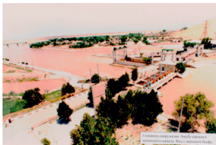
Headwork of Amubukhara pumping canal
