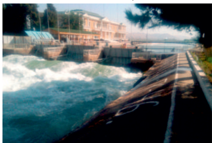
Vakhsh Main Canal at DP-46
