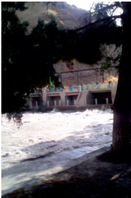
Tail-water of Dekhkanabad head intake structure
