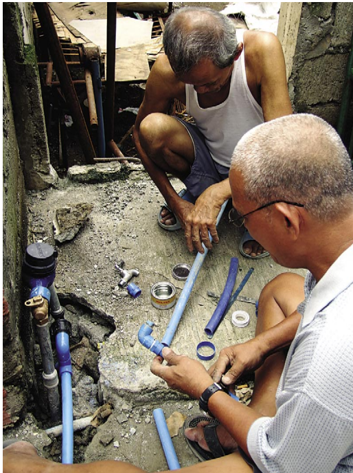
Installing metered pipelines in Manila's Alitaptap community
