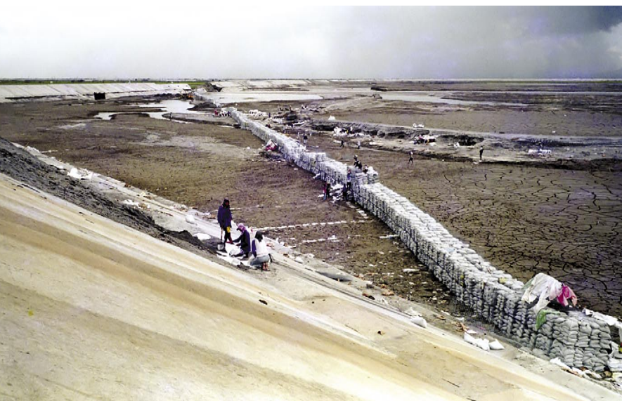
Mega Dike or the FVR dike in central Luzon being supported by sand bags.
