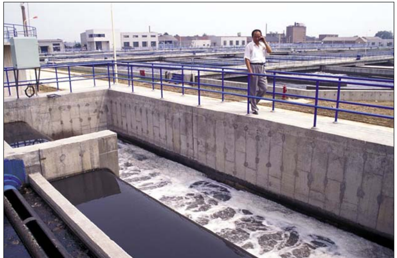
Inspecting Tangshan City Dongjiao Waterwaste Treatment Plant, People's Republic of China
