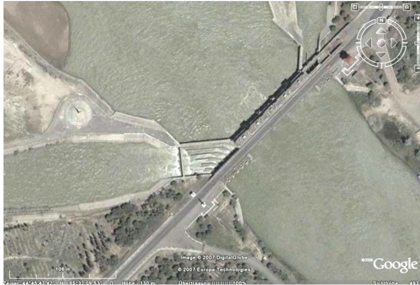
Figure 3.8 Reconstruction of LMC offtake regulator at Kzylorda barrage
