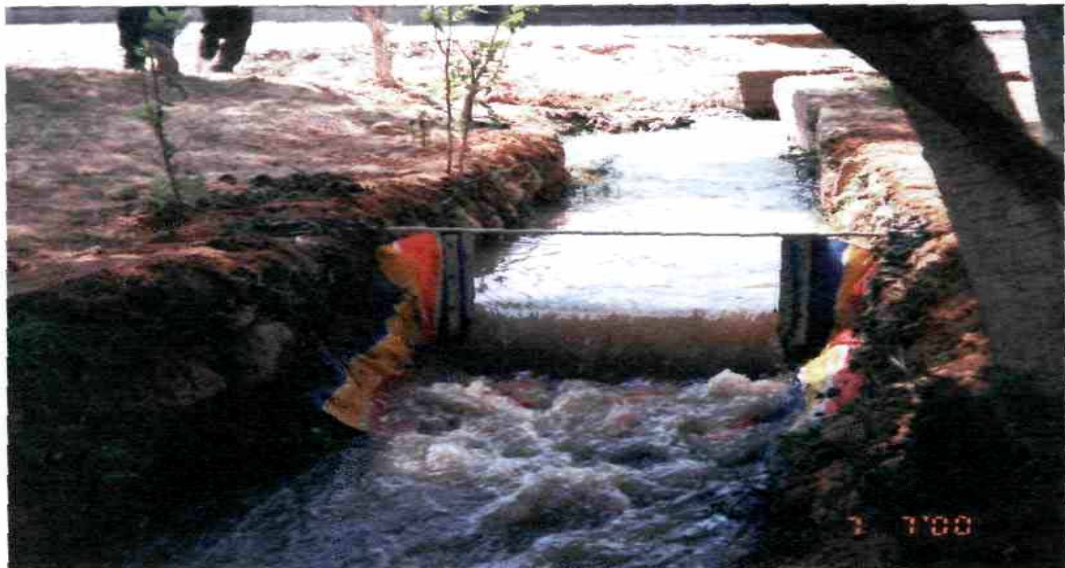
Transportable water spillway engineered by Sattarkulov.
