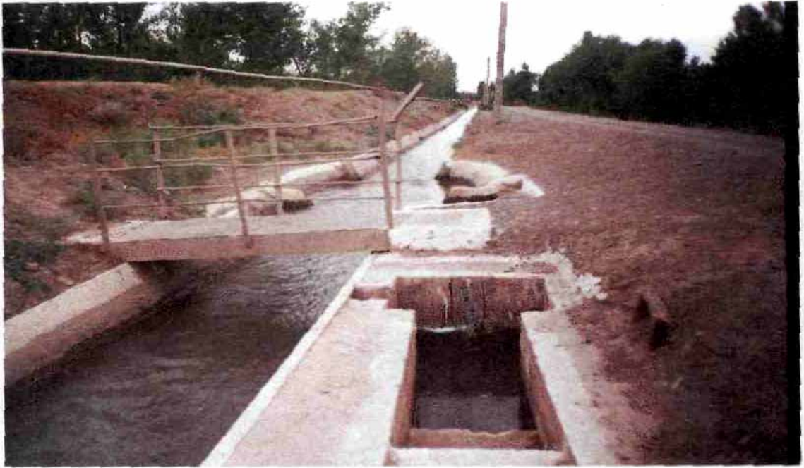
Hydrostation at flumed irrigation network.
