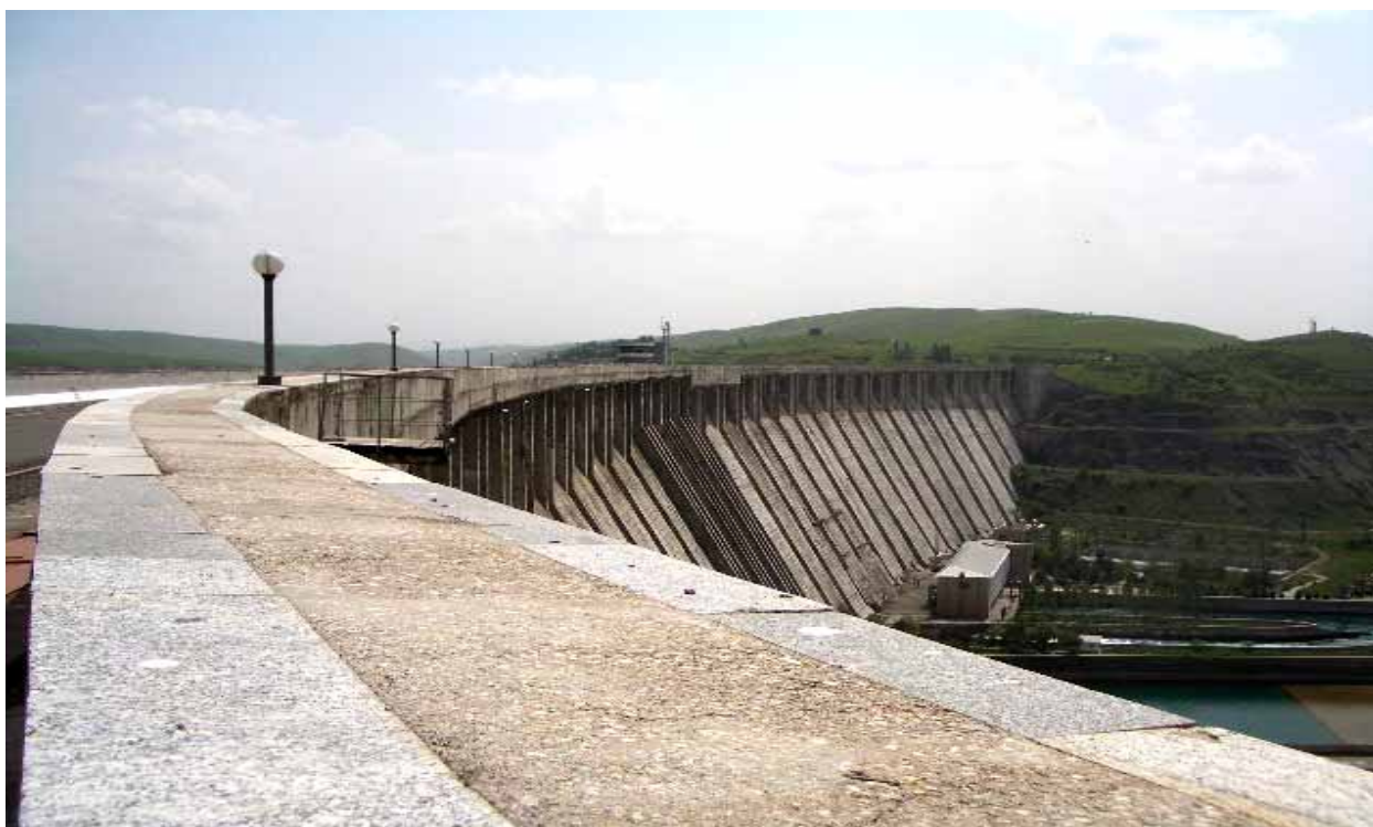
The Andijan water reservoir dam.
