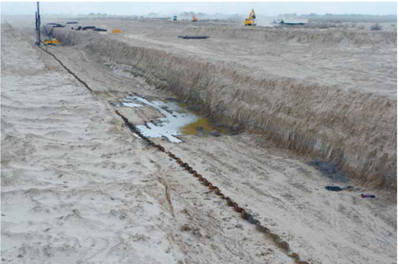
Spillway. Piling sheet pile into the base
