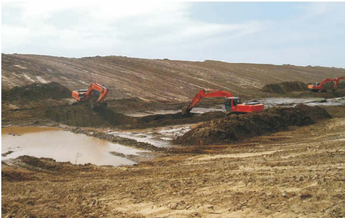
Figure 12. The Main South Drain Collector under construction in Karakalpakstan
