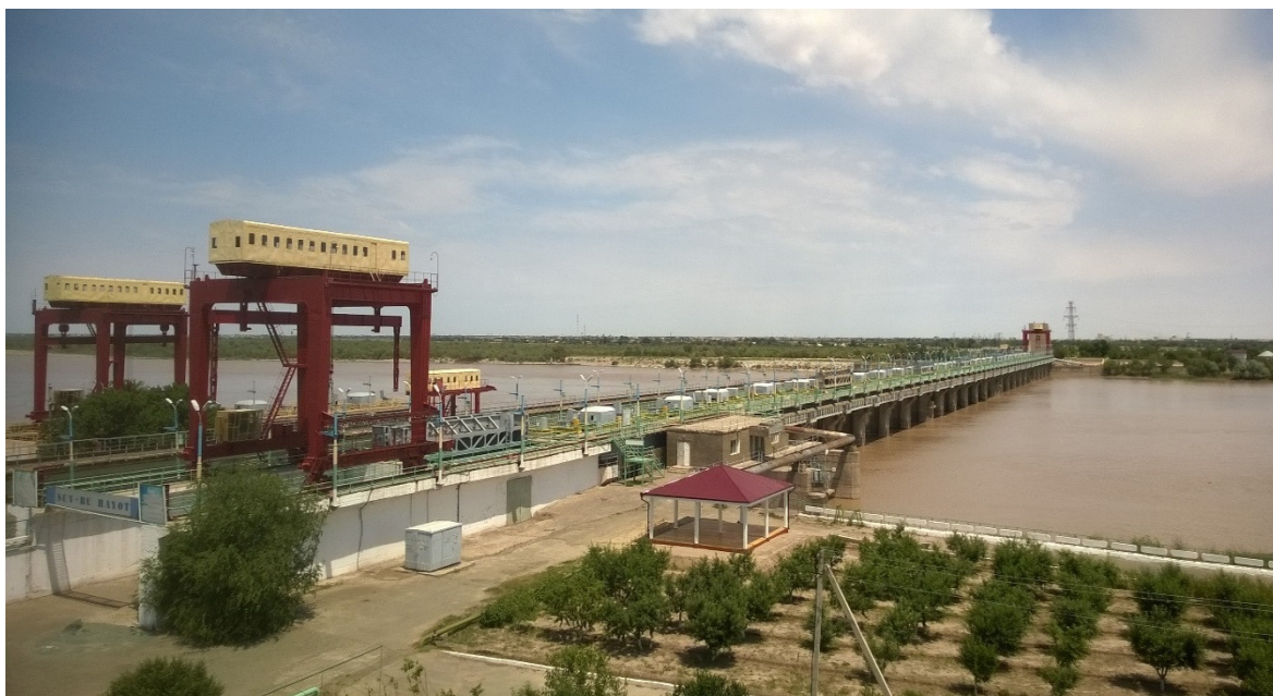
Figure 10. Takhiatash hydrostructure on the Amudarya river in Karakalpakstan (the biggest water weir in Central Asia completed in 1974) – capacity more than 11000 m 3 /sec
