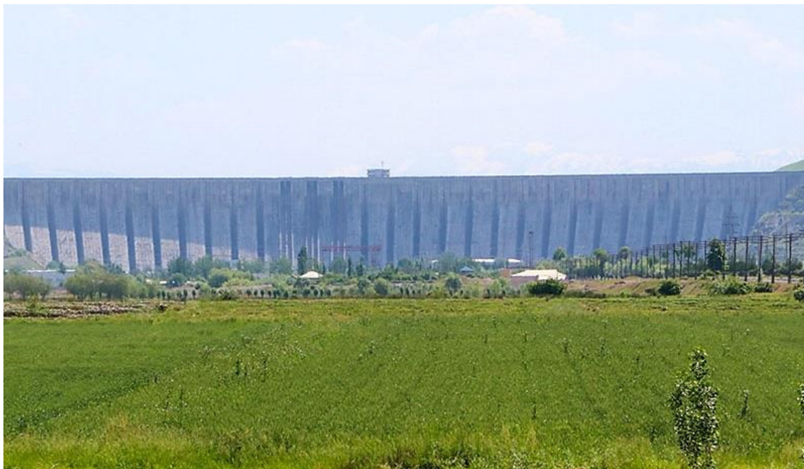
Figure 9. “Kampirravot” dam built on the Karadarya river. It was designed in 1962 and was completed in 1968-1982. The total length 1020 m. Dam is massive concrete with double buttresses-875 m. Maximum height 115 m.
