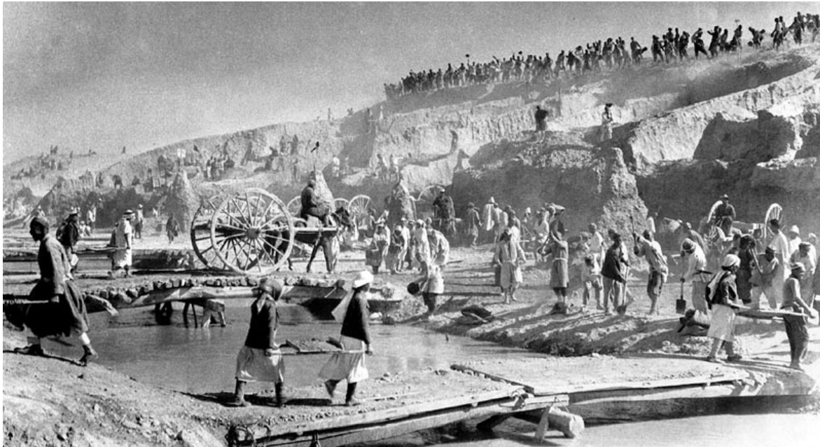
Figure 6. Thousands of dekhkans were mobilized for construction of the Great Fergana Canal in autumn of 1939 (discharge 100 m 3 /sec, length 270 km. It was constructed during the only 45 days by “khashar” method)
