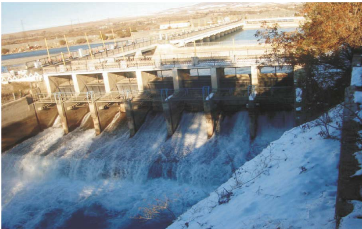
Figure 5. The Ravatkhodja Hydrostructure on the Zarafshan River
