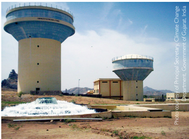
Water towers in Gujarat, India.
