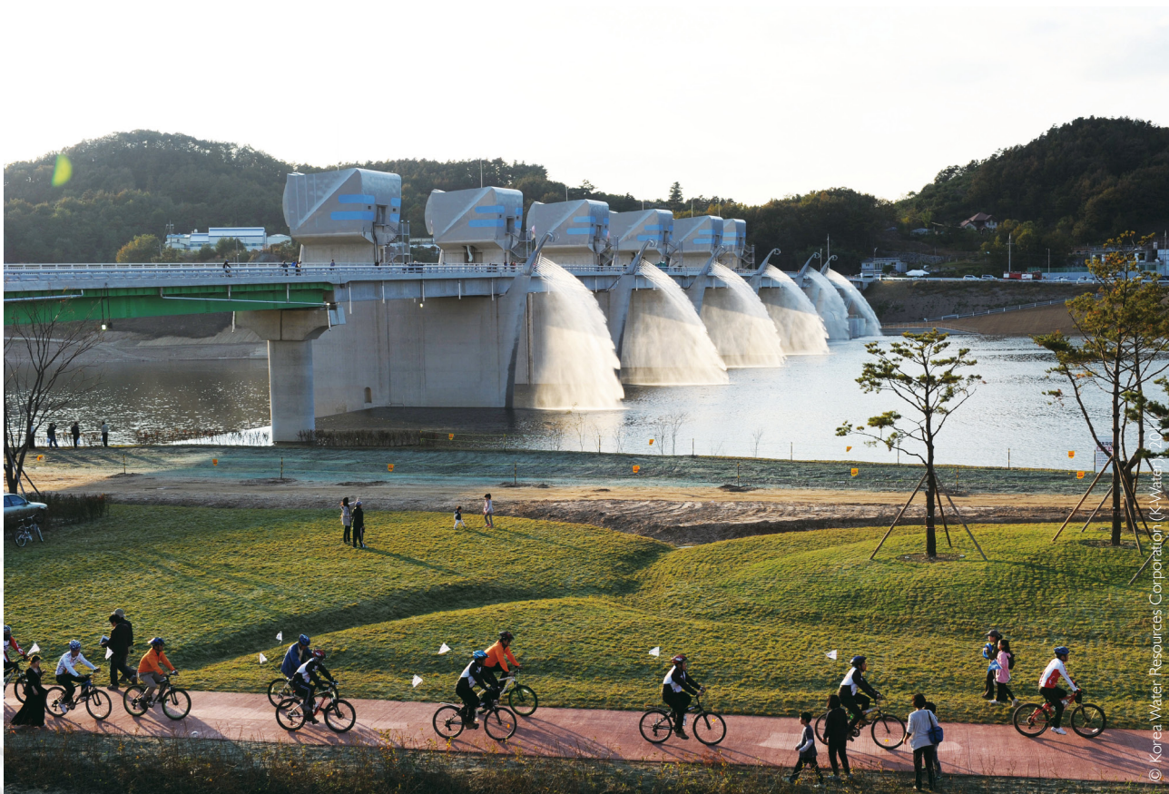
Four Major Rivers Restoration Project.
