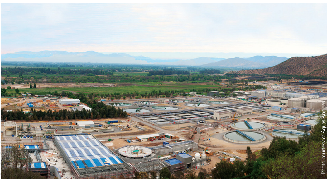
Treatment of wastewater at Planta Mapocho supports future green growth in the Santiago Water Basin.
