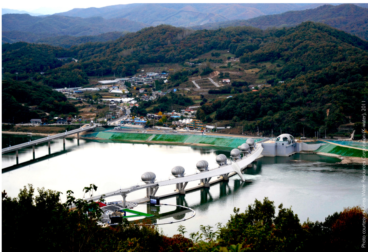
A new weir adjusts waterflow and helps store water needed during dry seasons in Ipo.
