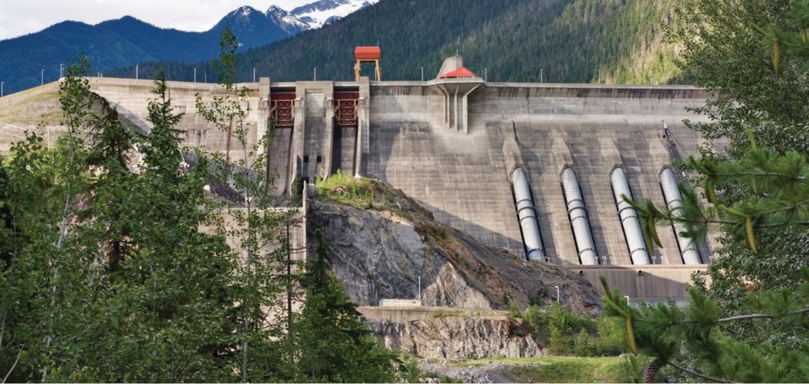
Revelstoke Dam, Columbia River Basin. © jmoor17/iStock.
