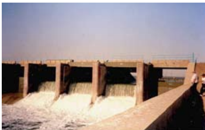
Figure 11. Spillway of new dike in the Berg strait in September 2006 (photo by L.Kuznetsov).
