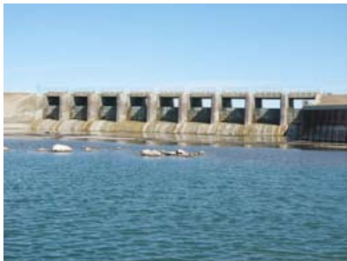
Figure 12. Spillway of new dike in the Berg strait in September 2007.
