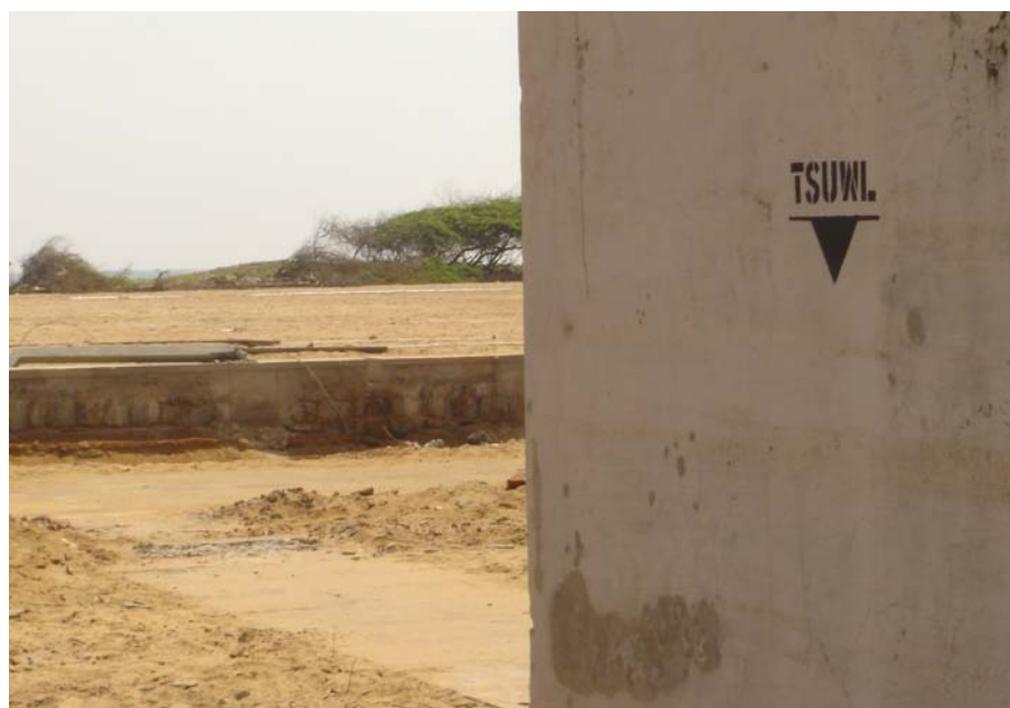
Figure 10.5.2 Water level mark showing height of tsunami intrusion
