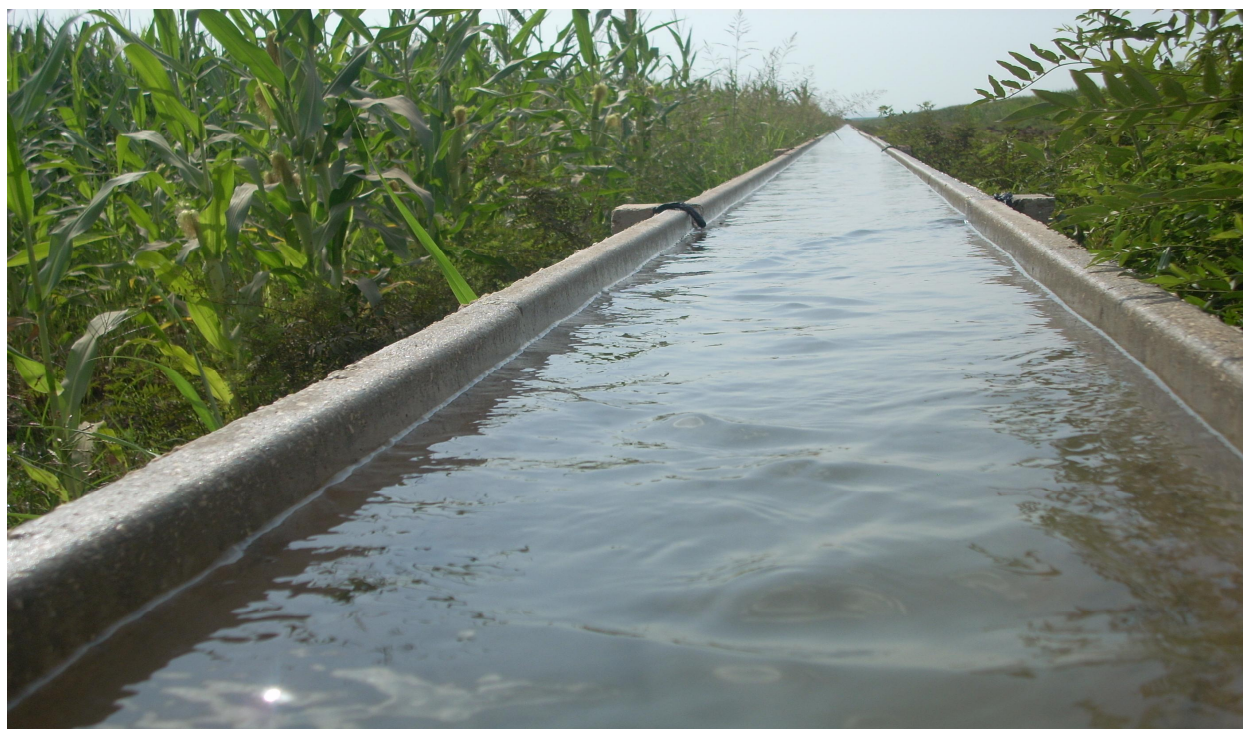
Figure 6.2 Secondary irrigation channels and siphon type irrigation of the maize fields, GAP
