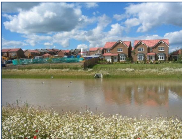
Figure 1.5.2 Example of a storage BMP: a retention pond (Photo credit: with kind permission of SUDSnet University of Abertay Dundee)
