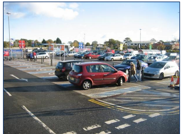
Figure 1.5.5 Example of an alternative surfacing material BMP: porous paving (Photo credit: with kind permission of SUDSnet University of Abertay Dundee)
