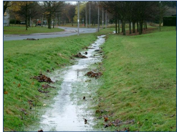
Figure 1.5.4 Example of a transfer BMP: a swale (Photo credit: with kind permission of SUDSnet University of Abertay Dundee)
