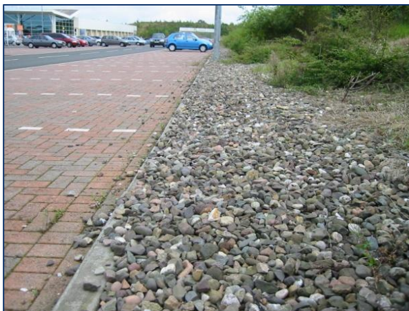
Figure 1.5.3 Example of infiltration BMP: a filter drain (Photo credit: with kind permission of SUDSnet University of Abertay Dundee)
