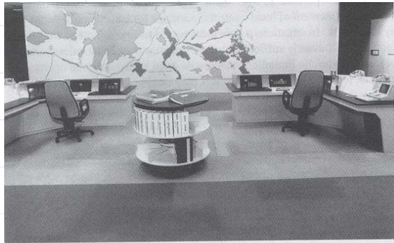
Fig. 5. Central Arizona Project SCADA System
