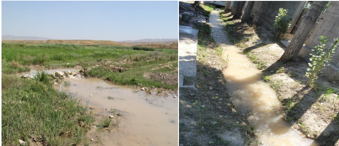
Figure 2. Water Canals in Bazar Korgon AA
