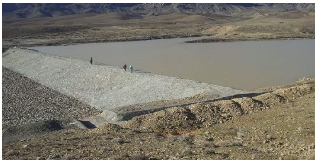
Figure 4. Recharge Dam in Kandahar Province (Stanikzai, personal collection, 2020).
