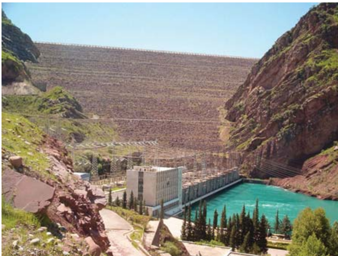
Figure 10. Nurek Dam on the Vakhsh River, Tajikistan (dam's height – 300m; water storage volume – 10500 mln. m 3 )
