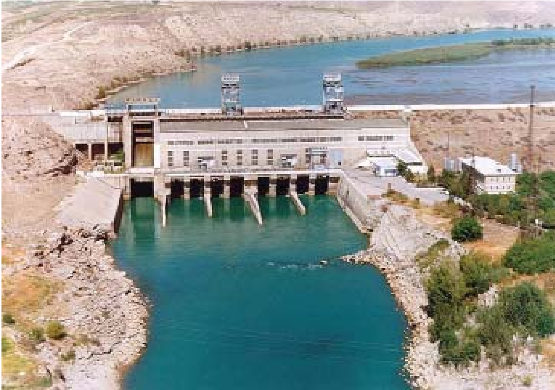
Figure 8. Uch-Kurgan Dam on the Naryn River, Kyrgyzstan (dam's height – 36m; water storage volume – 56,4 mln. m 3 )
