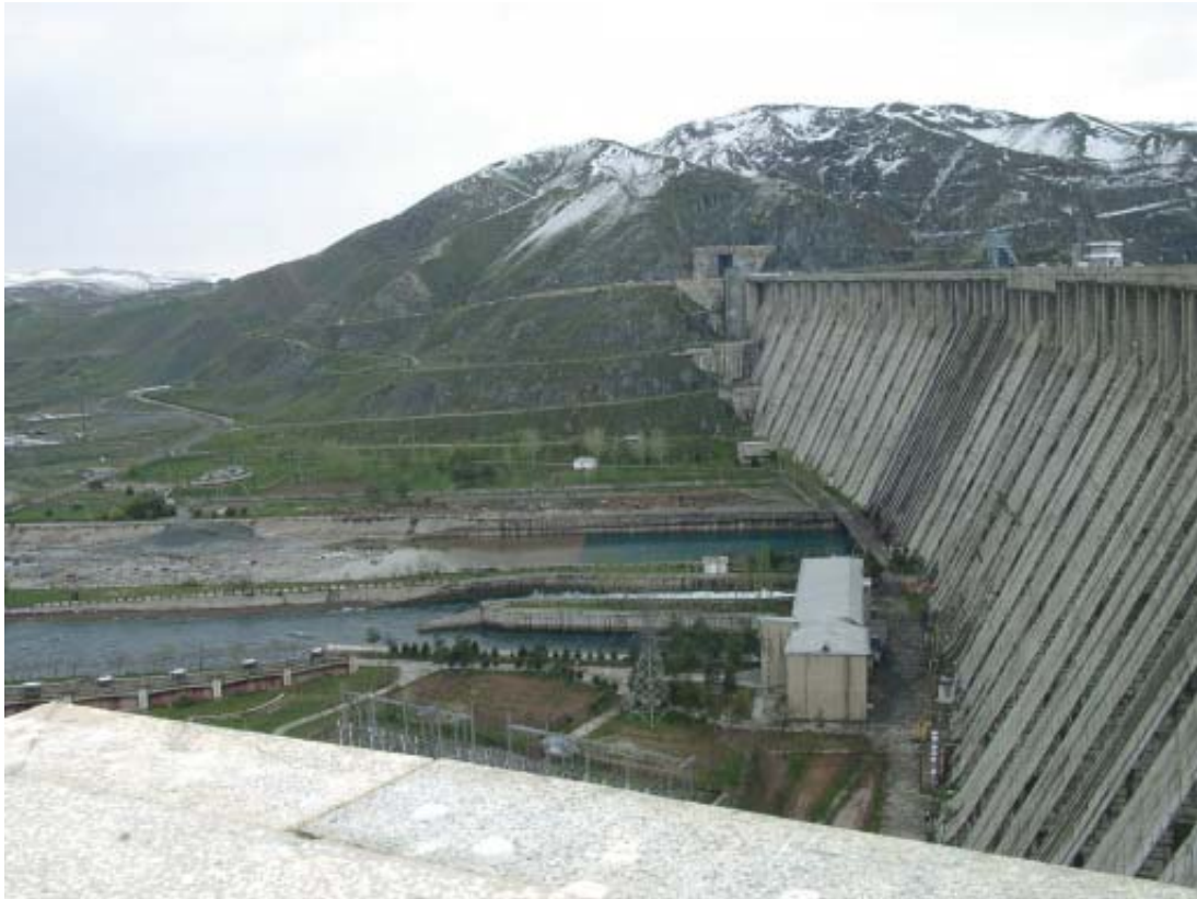
Figure 16. Andijan Dam on the Karadarya River, Uzbekistan (dam's height – 121m; water storage volume – 1900 mln. m 3 )
