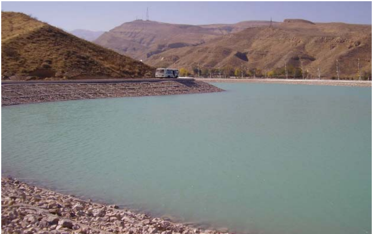
Figure 13. Pulikhatun waterworks on the Tedjen River, Turkmenistan (“Dostluk” dam's height – 78m; water storage volume – 1250 mln. m 3 )
