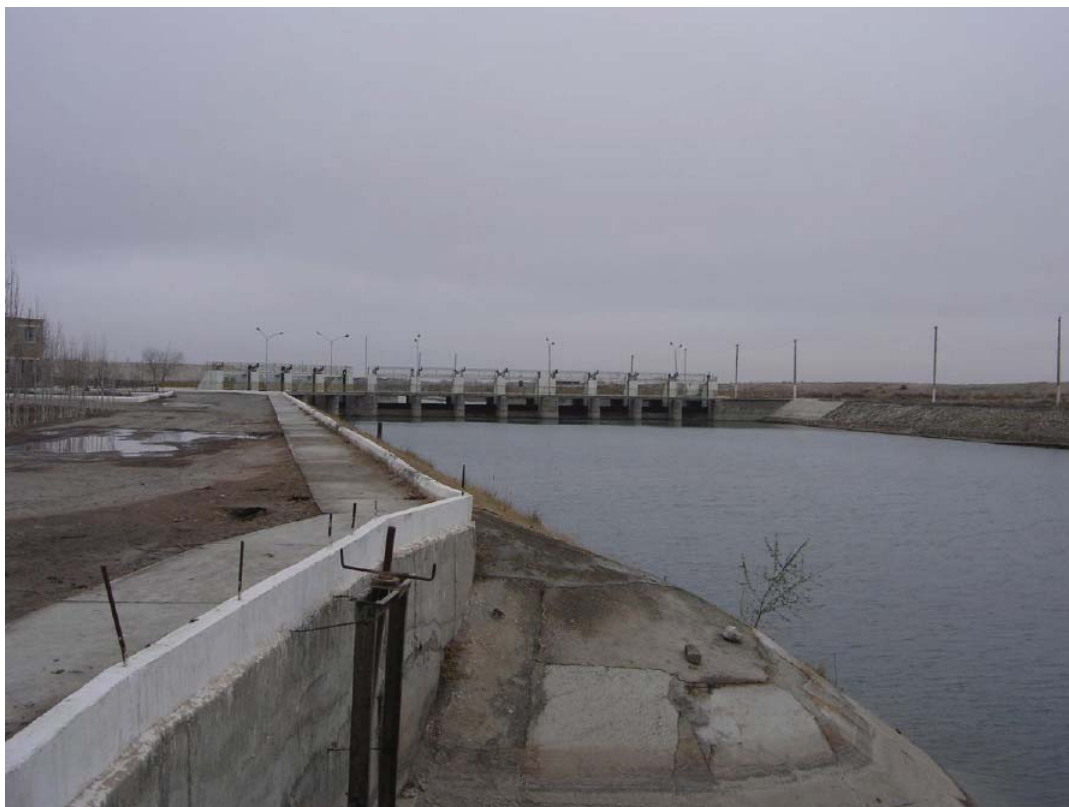
Figure 14. Oguzkhan Waterworks on the Karakum River, Turkmenistan (dam's height – 15m; water storage volume – 700 mln. m 3 )
