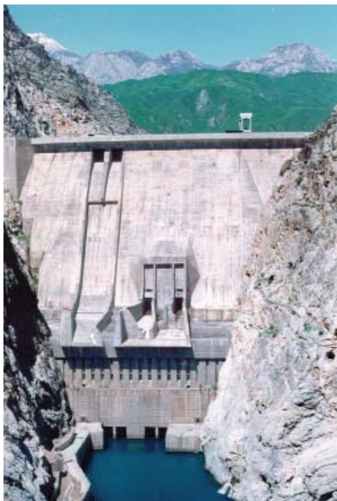
Figure 7. Toktogul Dam on the Naryn River, Kyrgyzstan (dam's height – 215m; water storage volume – 19500 mln. m 3 )
