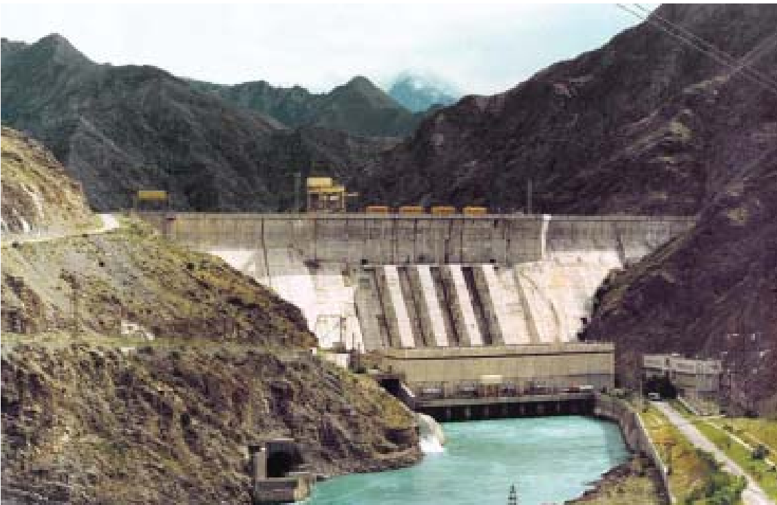
Figure 9. Kurpsai Dam at the Naryn River, Kyrgyzstan (dam's height – 113m; water storage volume – 370 mln.m 3 )
